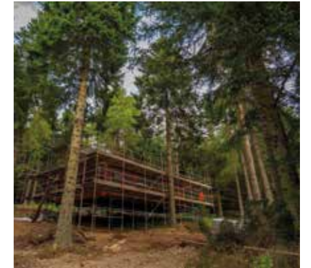
Cabin being erected within scaffolding.
