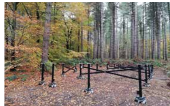
Low impact piling system for foundations, which do not disturb tree roots.
