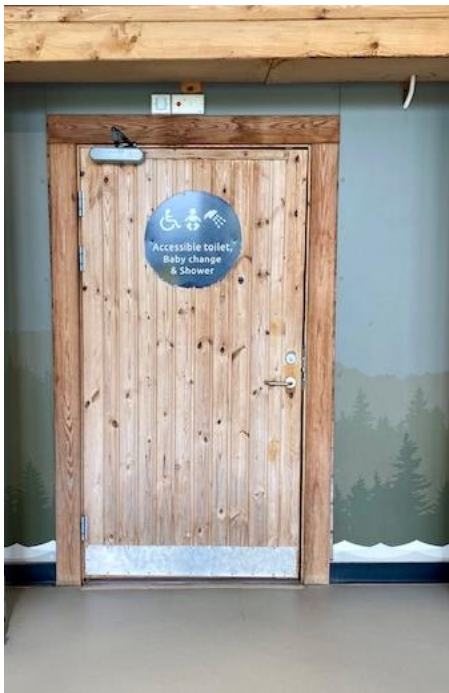
Entrance to accessible toilet
