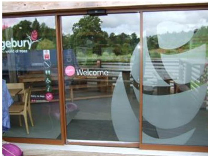
Automatic sliding door accessed from ramp and leads to the atrium, café, and toilets
