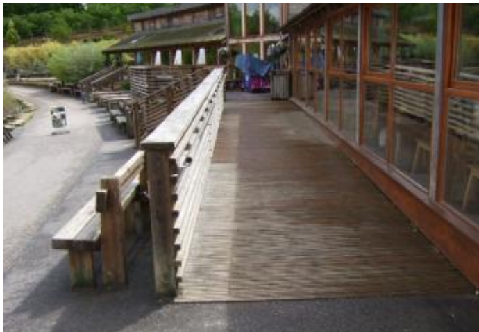
Ramp leading to atrium and cafe
