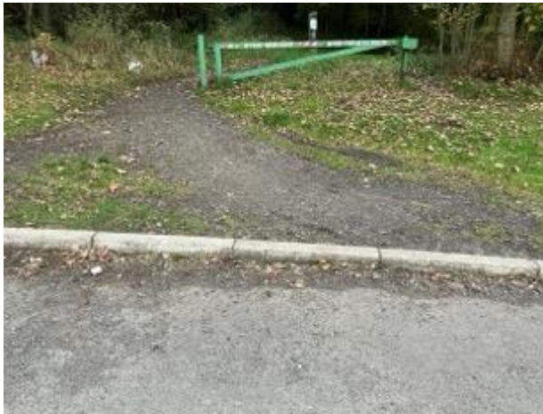
A lack of step-free access and lowered kerb onto the path from Marx Terrace joining Coal Tubs Way
