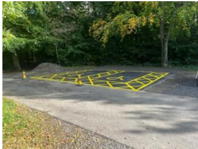
Two accessible parking bays are provided in the main car park
