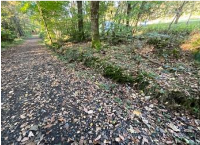
There are some shallow ditches on either side of the path in some areas.
