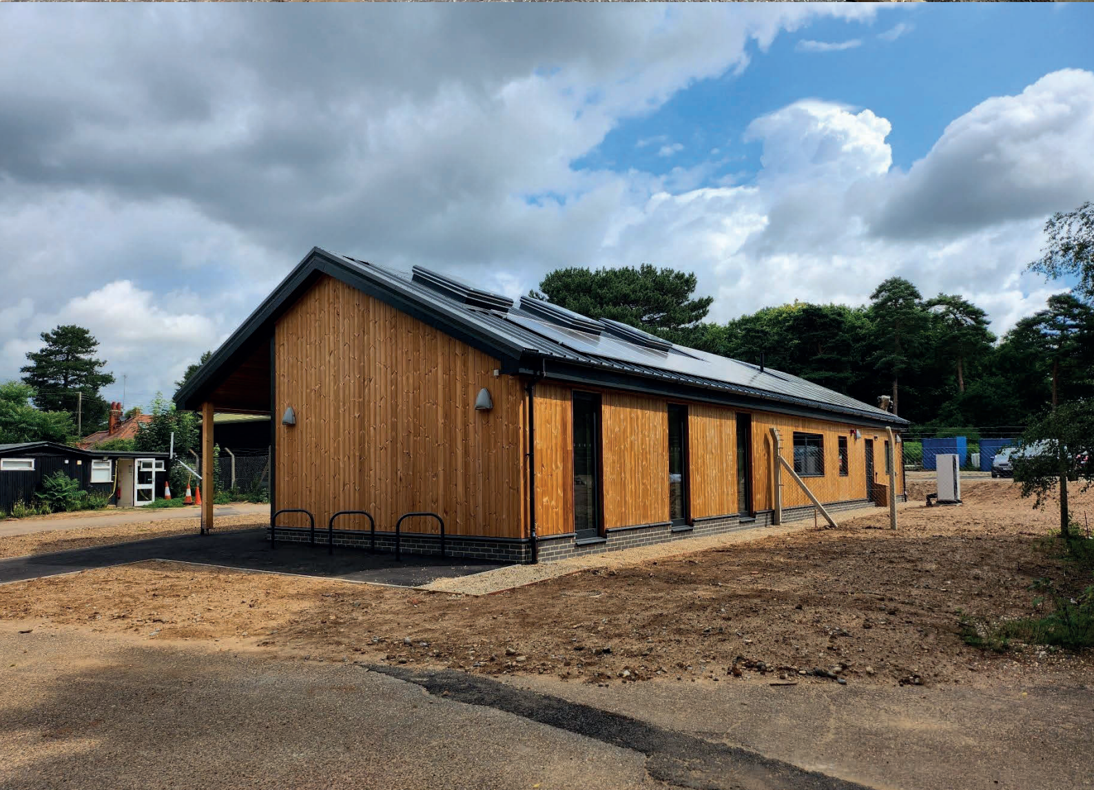
Demolition work taking place of the previous Tangham operations facility in East District.
