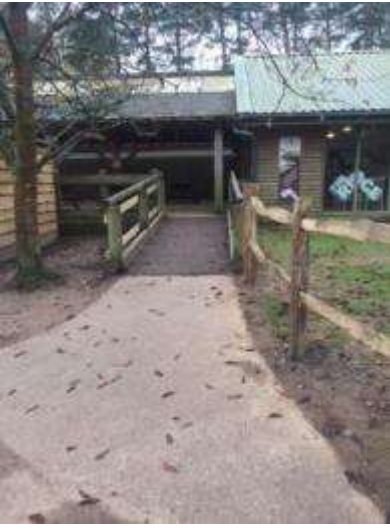
Ramp leading to The Ridge Cafe rear entrance and decking
