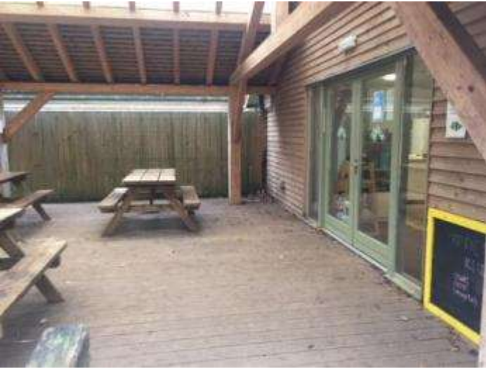
The Ridge Cafe rear entrance and decking area
