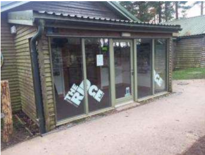
The Ridge Cafe Front Entrance
