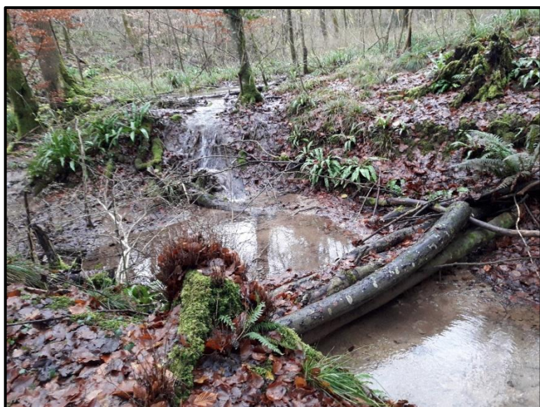
Figure 9 - Leaky dam in Kingscote Wood
