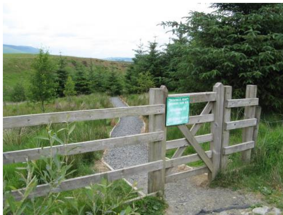
The new path & gate constructed by Troutbeck Caravan Park
