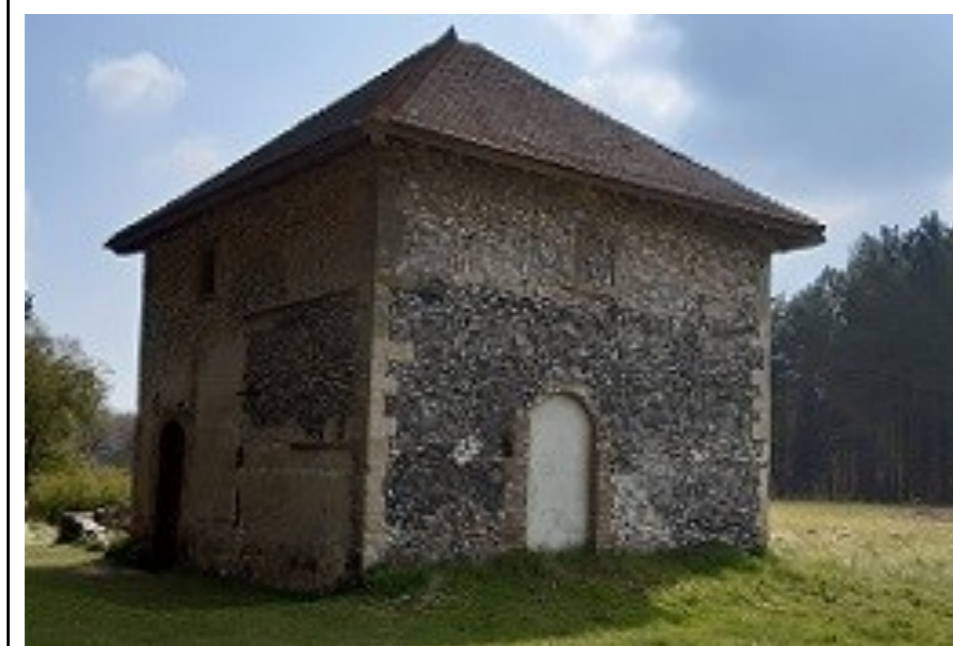
Mildenhall Warren Lodge looking south-east. Photo: K Truscoe (April 2021)
